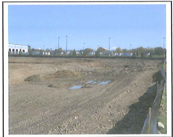
One of the stormwater basins rough graded.
