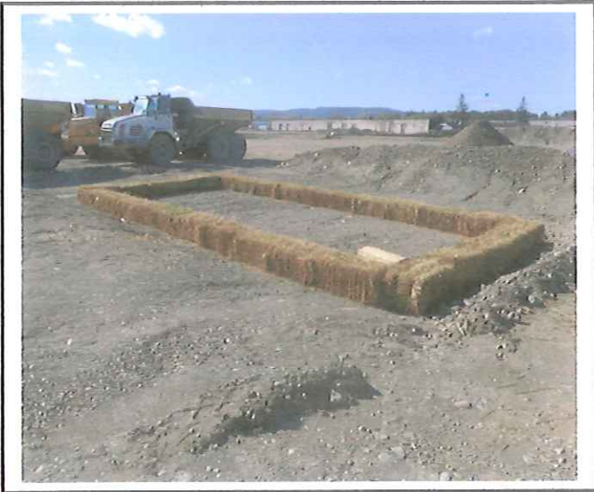
Beginning of concrete washout area.
