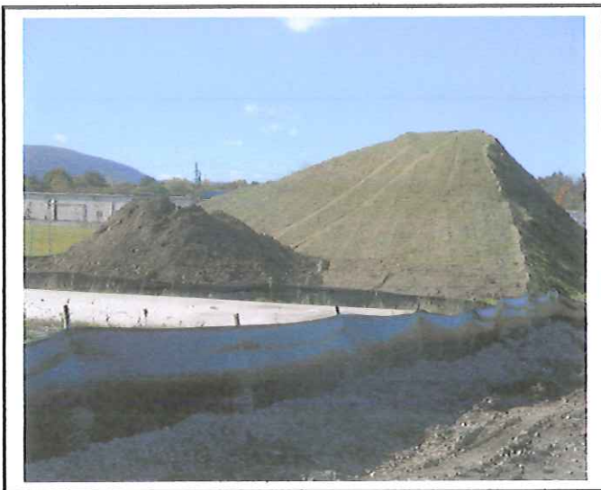
Topsoil pile has been seeded and is growing grass.
