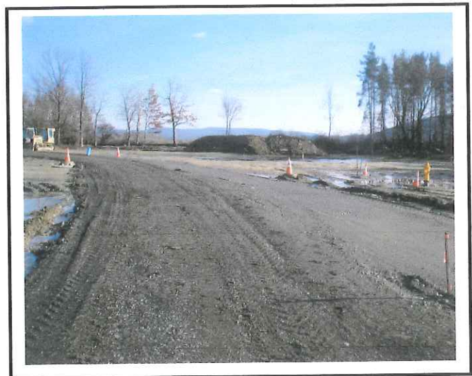
Stockpiles that are actively being built.
