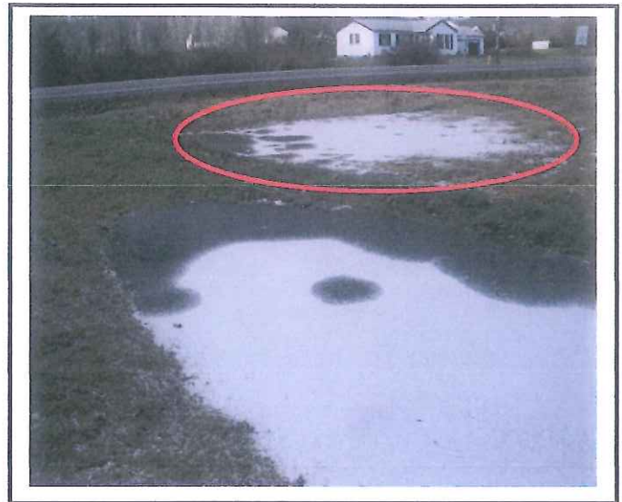
VOS BCD: Area near Hickory Grove Road where stormwater left the site through a low spot in the stormwater swale.
