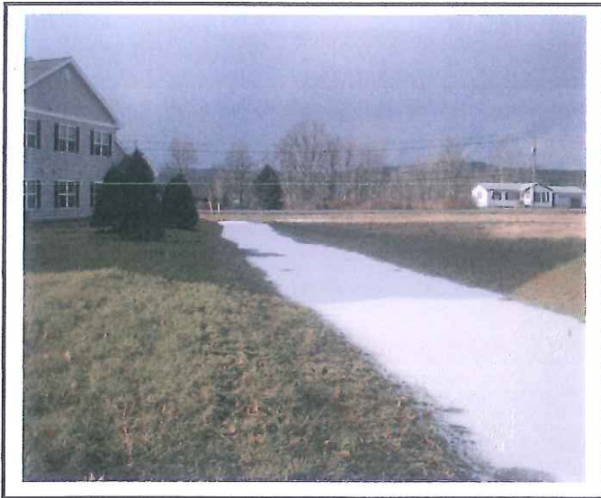
Vegetated Open Swale (VOS) BCD. Standing/frozen water present.
