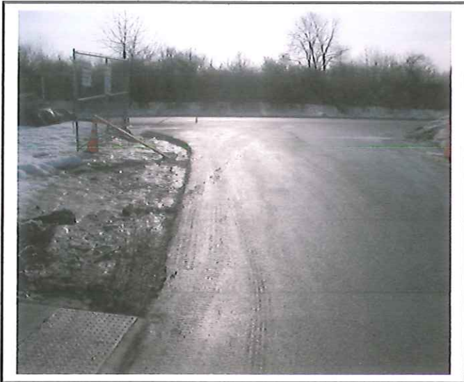
Entrance and exits are clear of mud being tracked off site.
