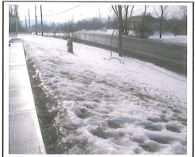
Open areas require stabilization once snow melts.
