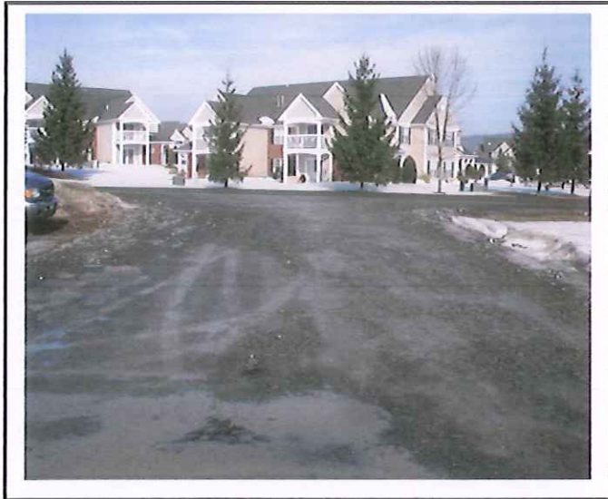
Construction Entrance is okay now but will need to be monitored for tracking into the road during "mud season".
