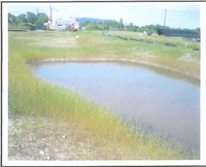
Stormwater forebay is holding water.
