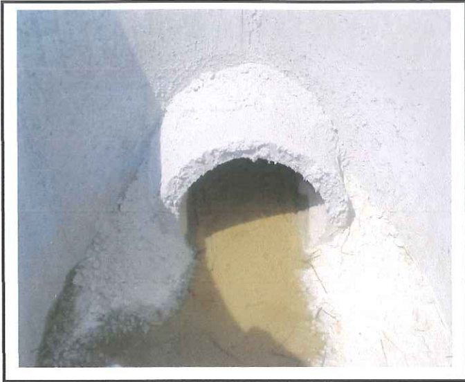
Outlet pipe has been grouted.
