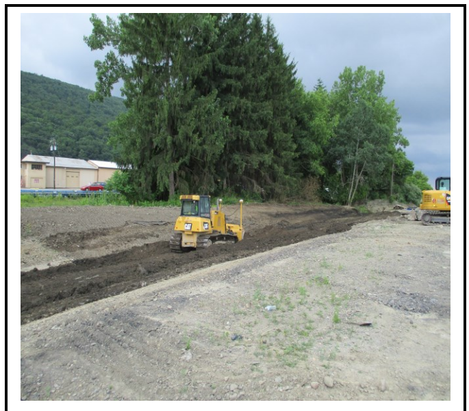
Grading of drainage swale occurring at time of inspection.
