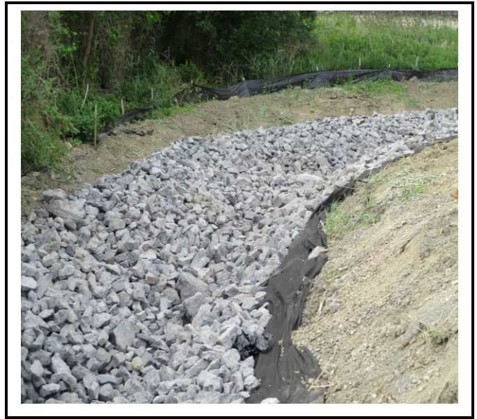
Rock lined swale being installed at time of inspection.
