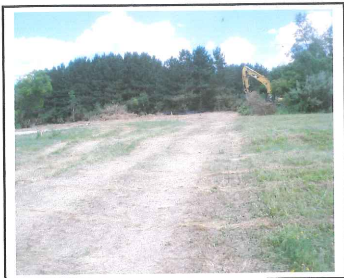
Area being excavated for fill.
