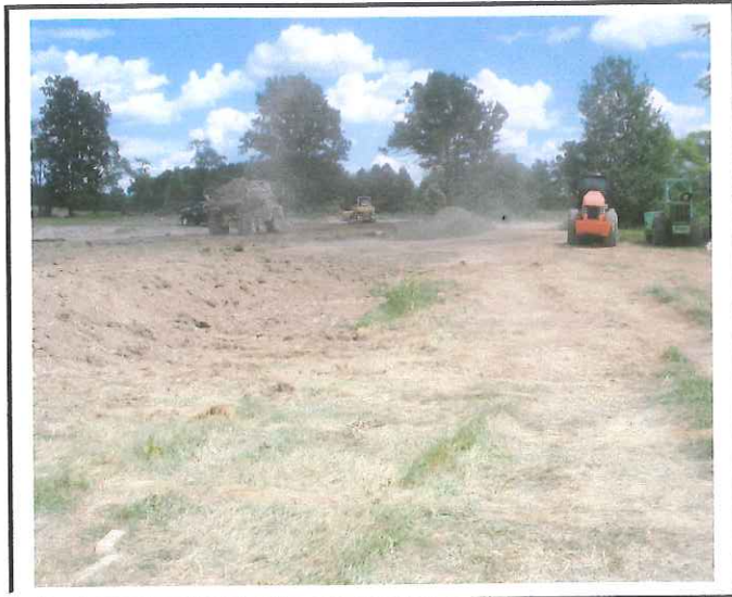
Project road construction.
