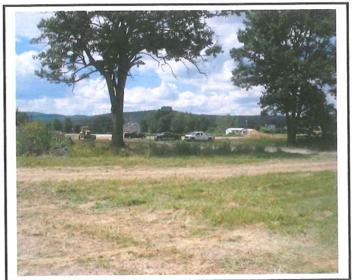
Active work area.
