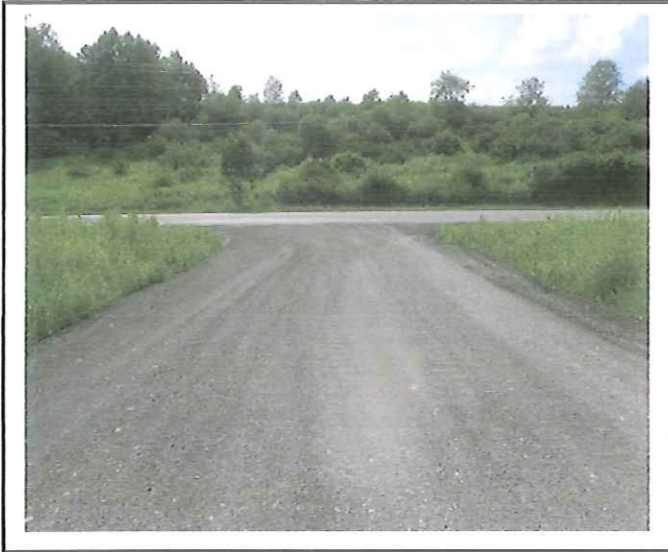
Construction entrance is clean and clear of debris.
