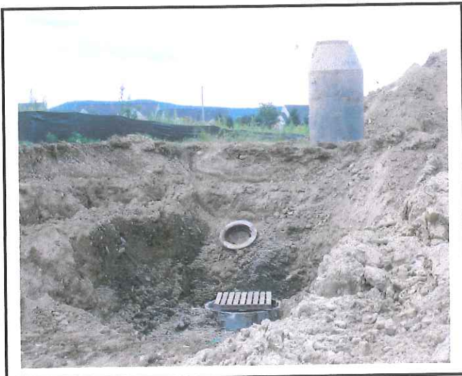
Sanitary tie in.
