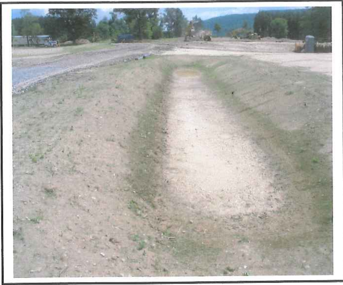
Infiltration trench F1.
