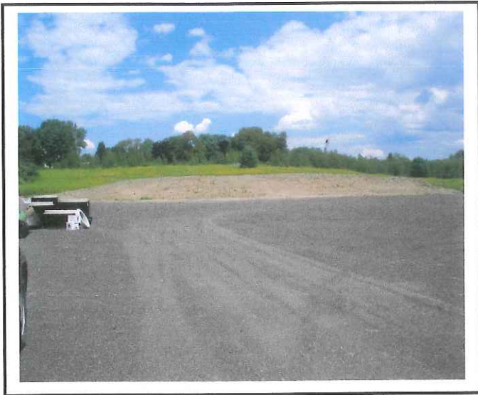
Contractor staging yard and stockpile area- the stockpile has been hydroseeded.
