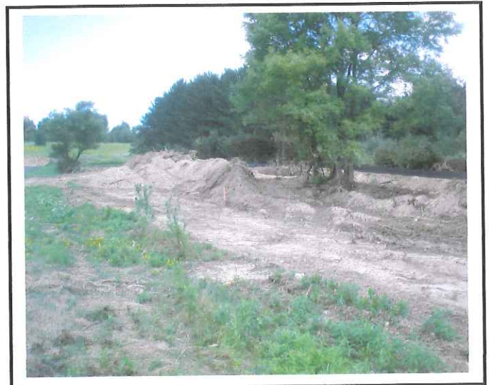
West side of construction area where active filling is occurring.
