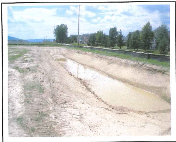
Infiltration F3- holding lots of water.
