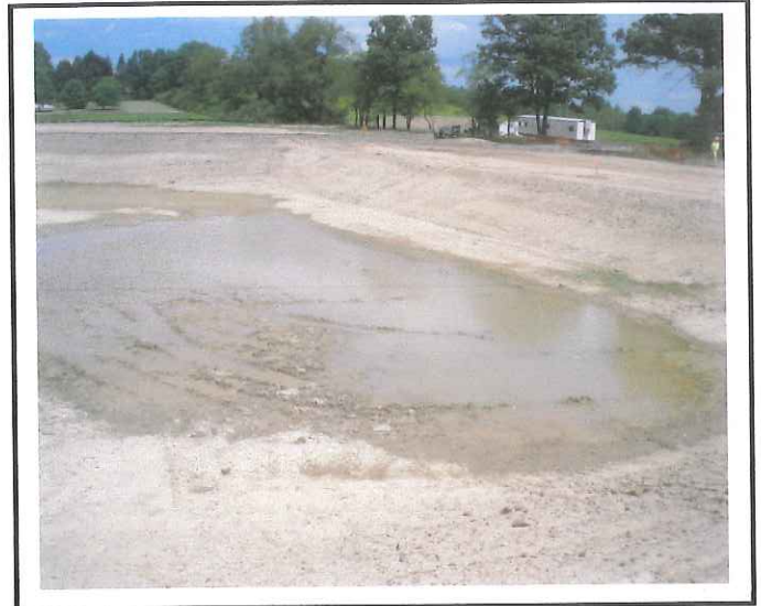
Stormwater pond 1A.
