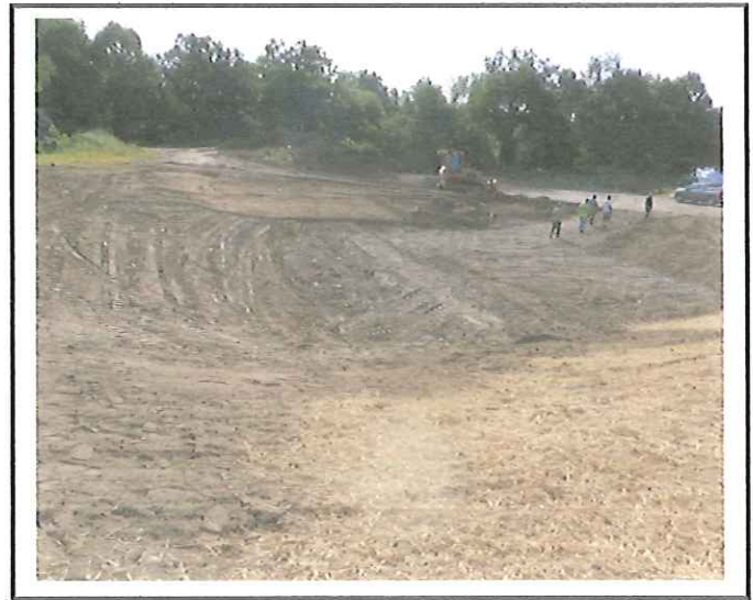
Scratched in infiltration basin.
