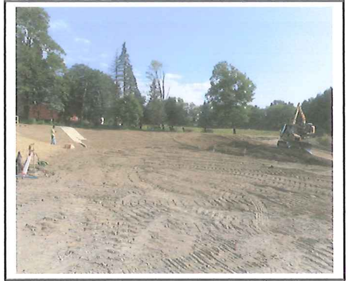
Topsoil being spread on side slope of infiltration basin.
