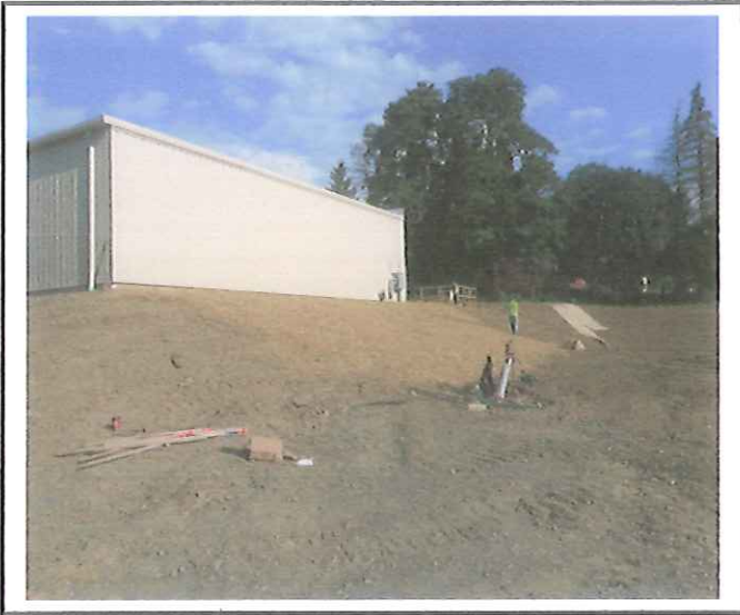
Slope behind building was being stabilized at time of inspection.
