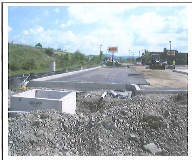
Silt fence remains in the back of property.
