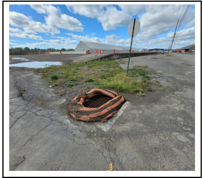
Compost sock inlet protection at most south end of building requires replacement
