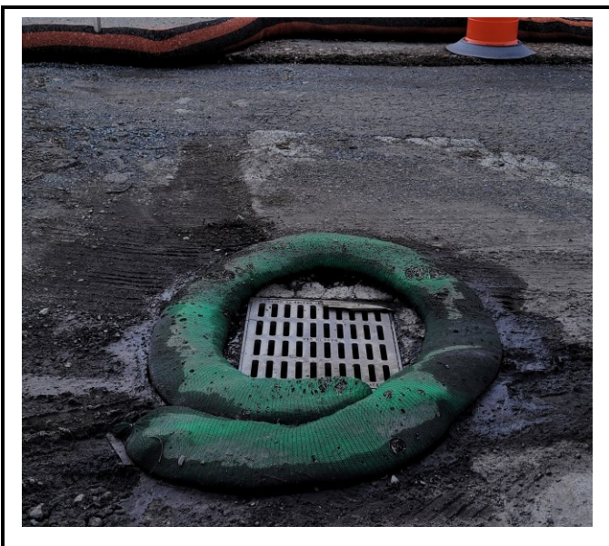
Inlet protection cannot be driven over. Anywhere that inlet protection has been flattened to the point of not providing protection requires replacement
