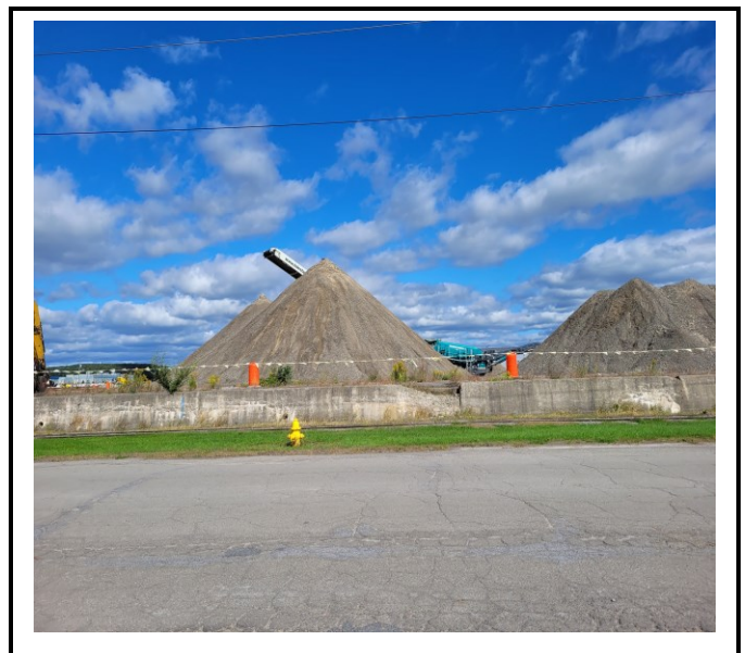
Stockpiles of finer materials do need sediment control around them.
