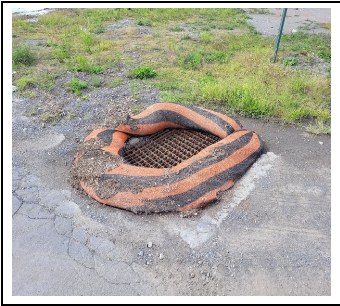
Compost sock inlet protection at most south end of building requires replacement
