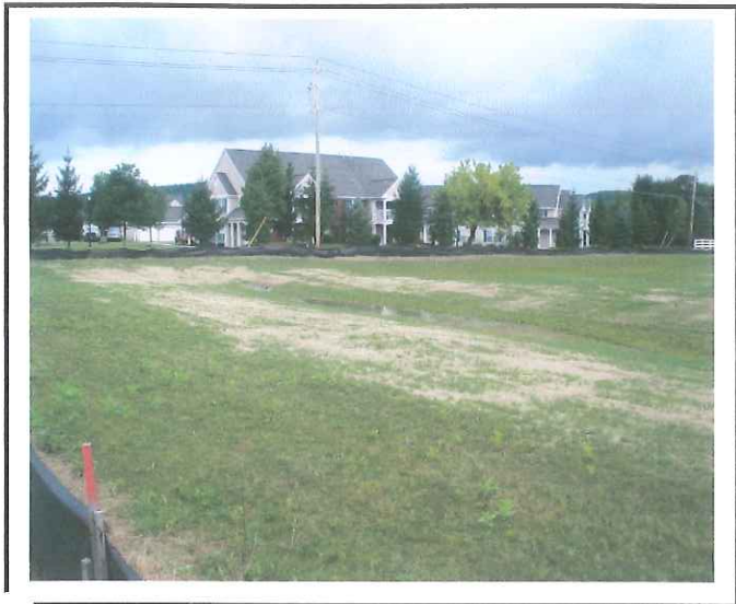
VOS F4 holds water and is not establishing vegetation easily.
