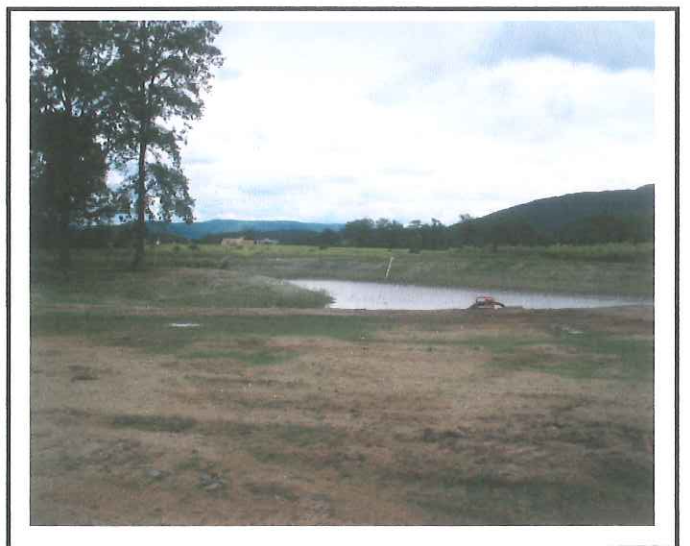
Back pond being pumped down.
