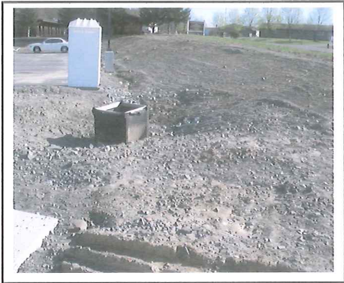
Erosion is occurring in the swale next to Biltmore drive and Building G. Light posts may be causing. Swale needs re-grading and stabilization.
