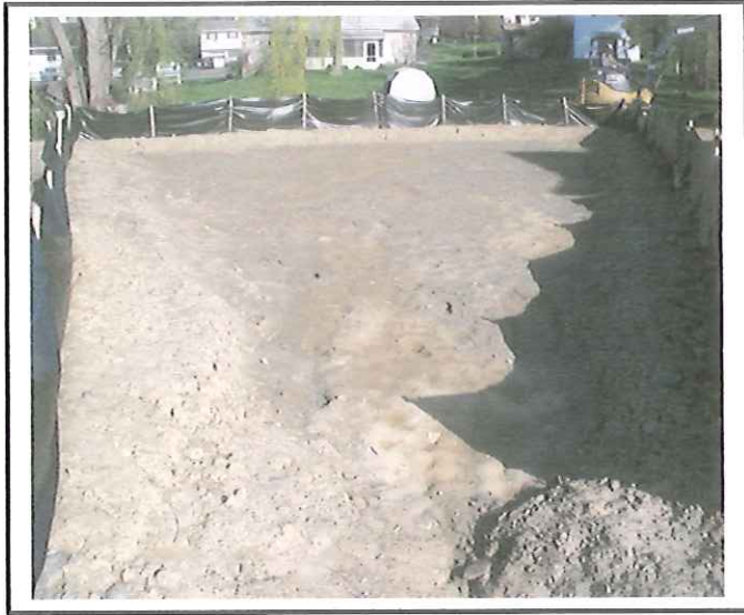
Rain Garden 1 is partially installed but sediment is getting into it. We will want to see the soil media prior to its installation.
