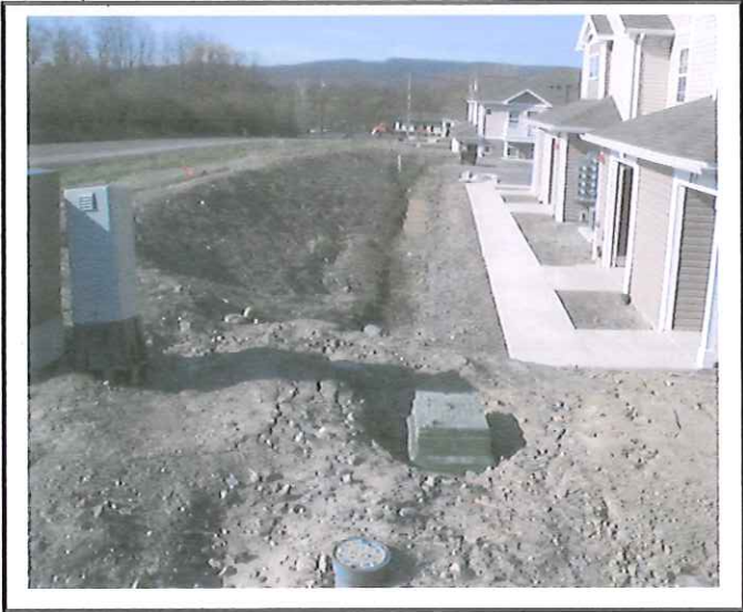
Many steep slopes around the buildings have yet to be topsoiled and stabilized.
