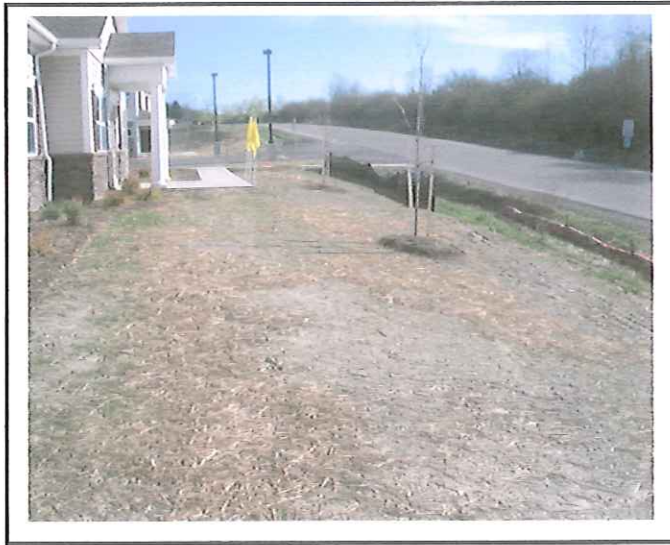
Areas around the Community Building and building C are not growing grass. These areas do not look like they will be suitable for growth-re-grading is necessary.
