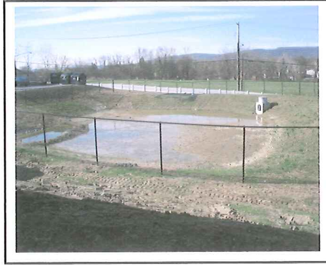
Pond will need to have sediment cleaned out of it prior to close out. Permanent stabilization is required. 1 foot berm pond and Building D has not been constructed.
