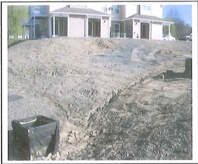
Swale in front of Building E is eroded and not stabilized.
