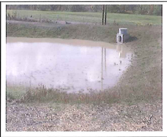
Stormwater pond is being utilized as a sediment trap.
