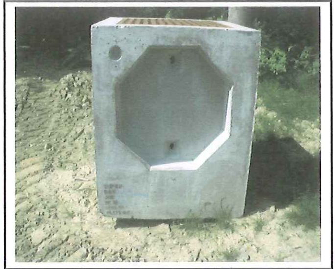
New pond outlet structure.
