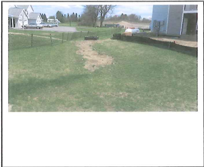
Swale will need to have sediment removed prior to final close out.
