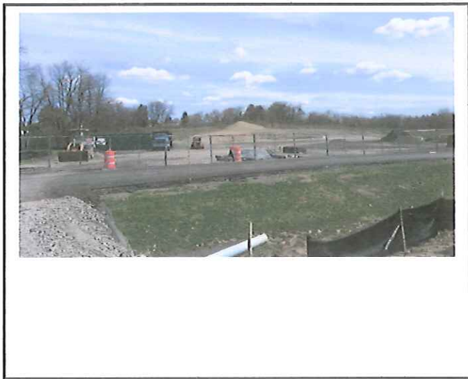
Stockpile in contractor yard needs to be seeded and mulched.
