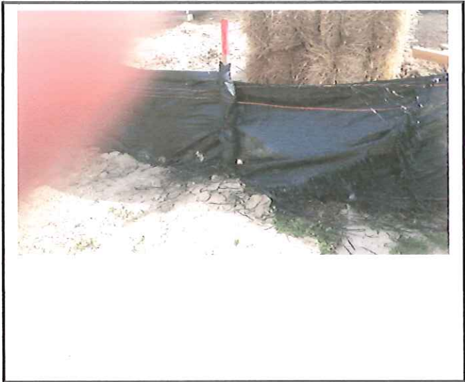
Silt fence requires repair
