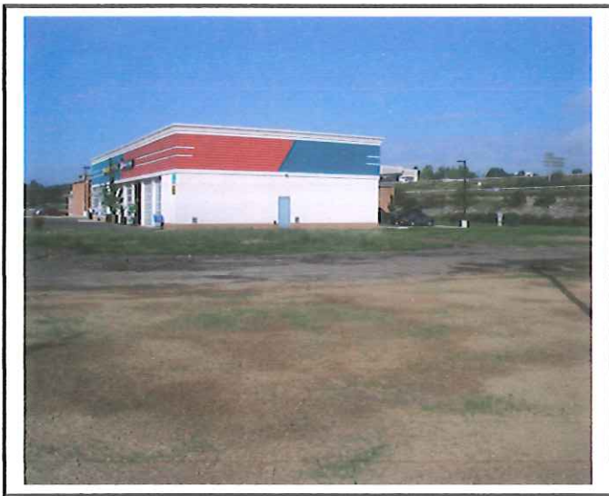
Area covered in milled asphalt that needs to be brought back to original condition.
