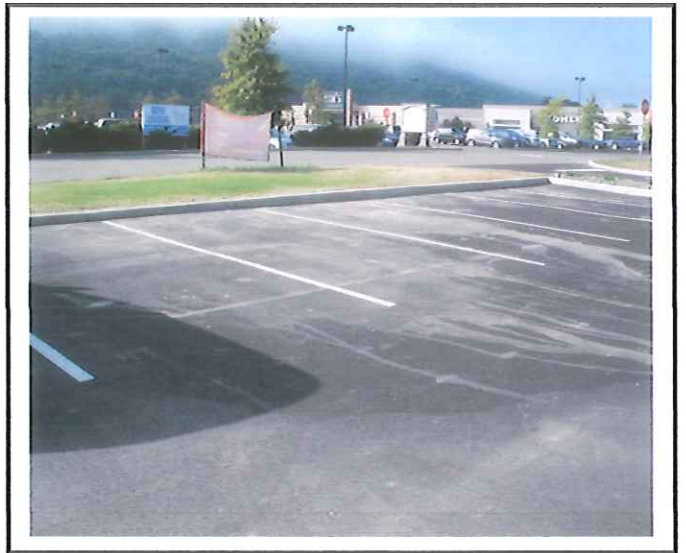
Sediment mixed with stormwater is flowing over concrete curbs into parking area. Soil does have hydro seed applied but minimal grass is growing.
