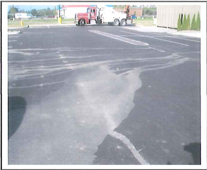
Sediment mixed with stormwater is flowing over concrete curbs into parking area. Soil does have hydro seed applied but minimal grass is growing.
