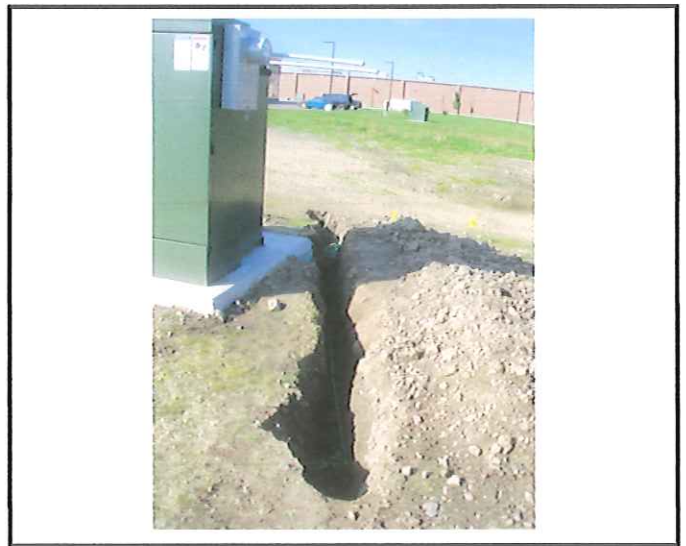
Trench open still.
