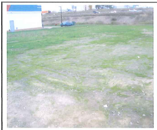
Area where asphalt millings were placed and have not been removed.
