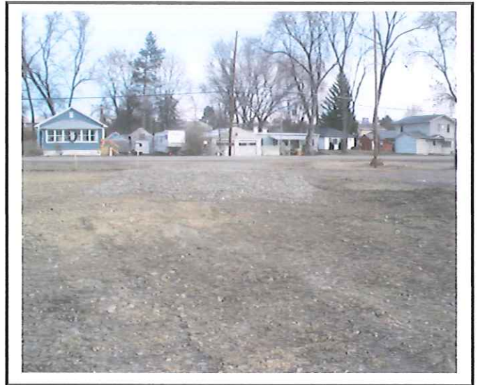
Construction entrance (2 nd ) installed.
