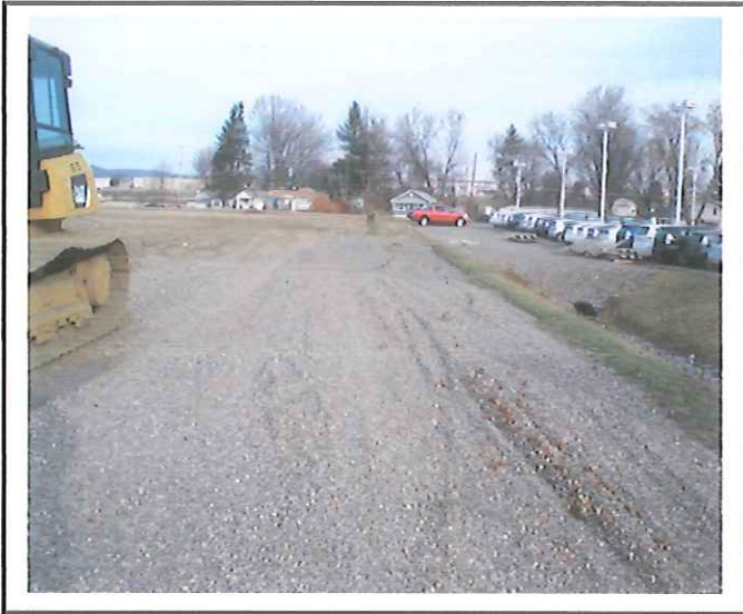
Construction entrance installed
