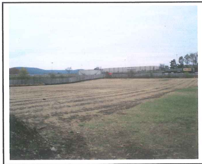
Overflow parking area has been graded and stabilized.
